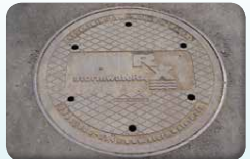
Clara maintenance manhole
